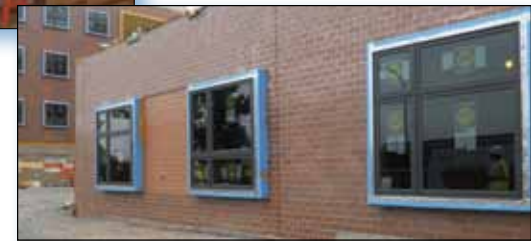
Windows in the ventilator unit
